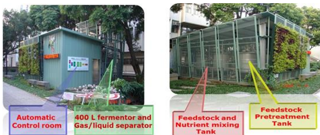
Figure 1. The world's first pilot plant for biohydrogen production on the campus of Feng Chia University, Taiwan.
