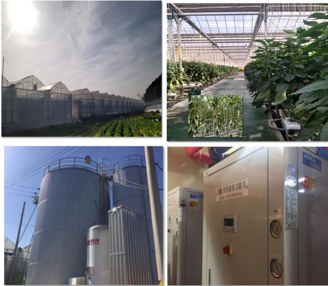
Fig.1. (Above) A view of the farm's geothermal facility, (Below) Heat storage tank and geothermal heat pump facility of the farm
